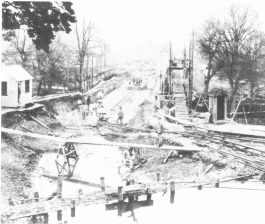
Repairs to the aqueduct on the Montgomeryshire Canal at Berriew, c. 1880.
